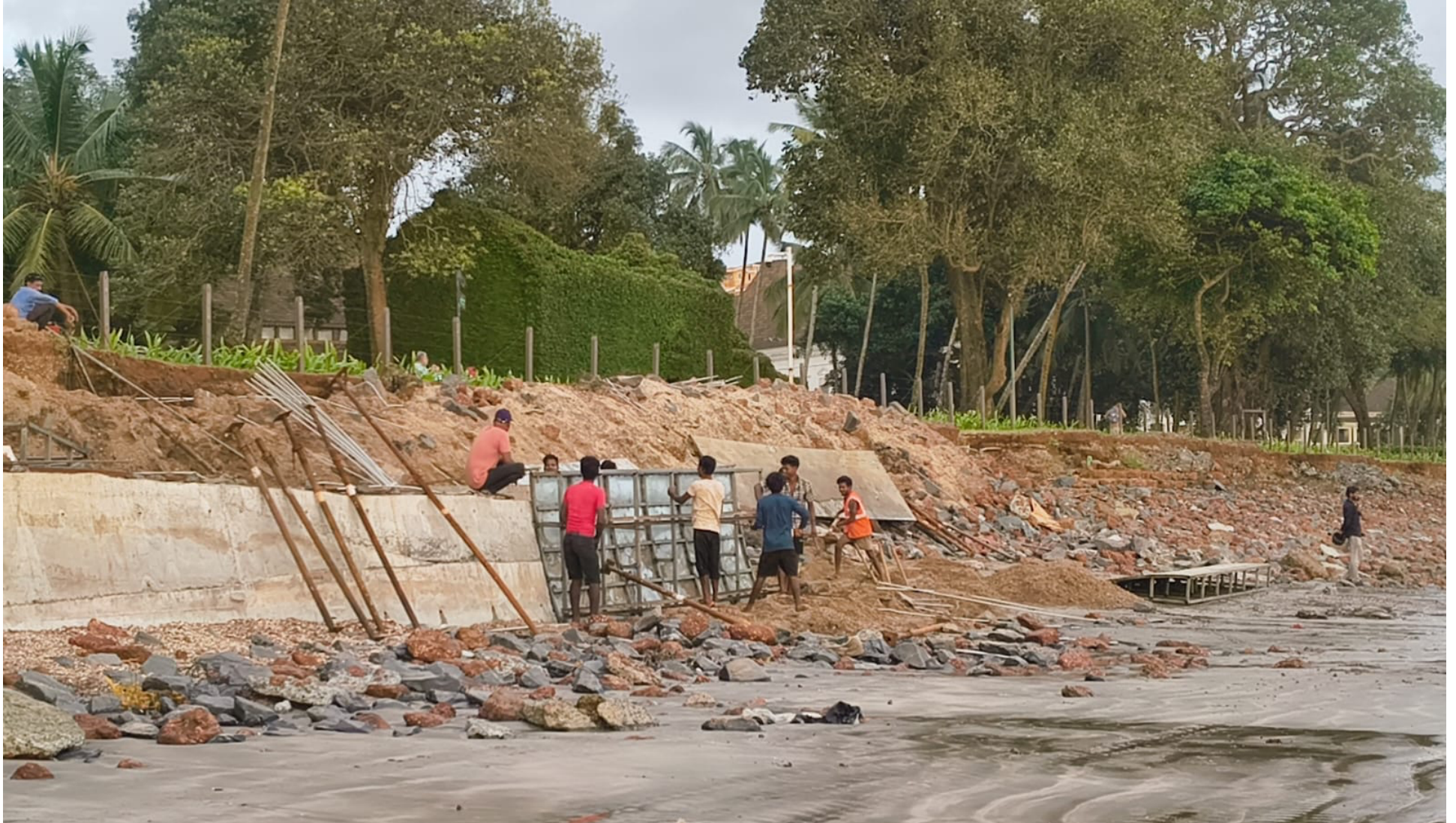
Latest pictures of the ongoing construction work dt. 25.08.2025
