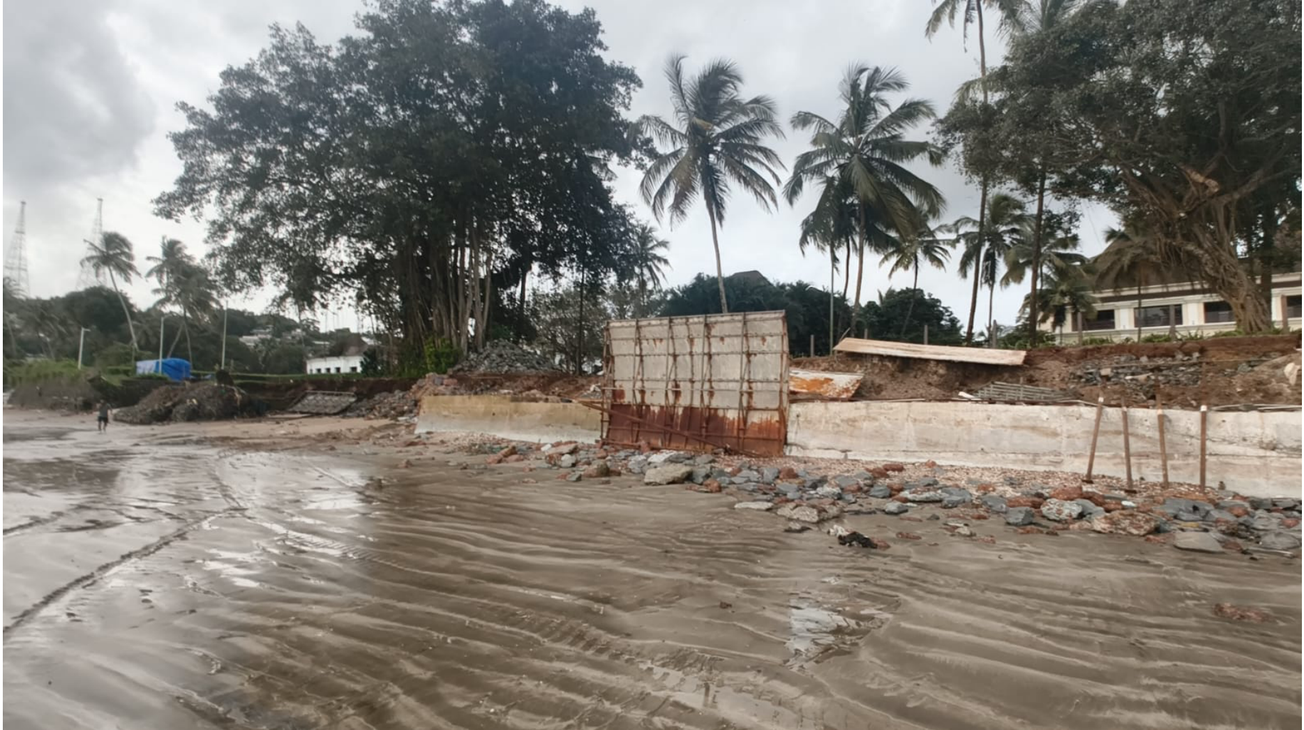
Latest pictures of the ongoing construction work dt. 26.08.2025
